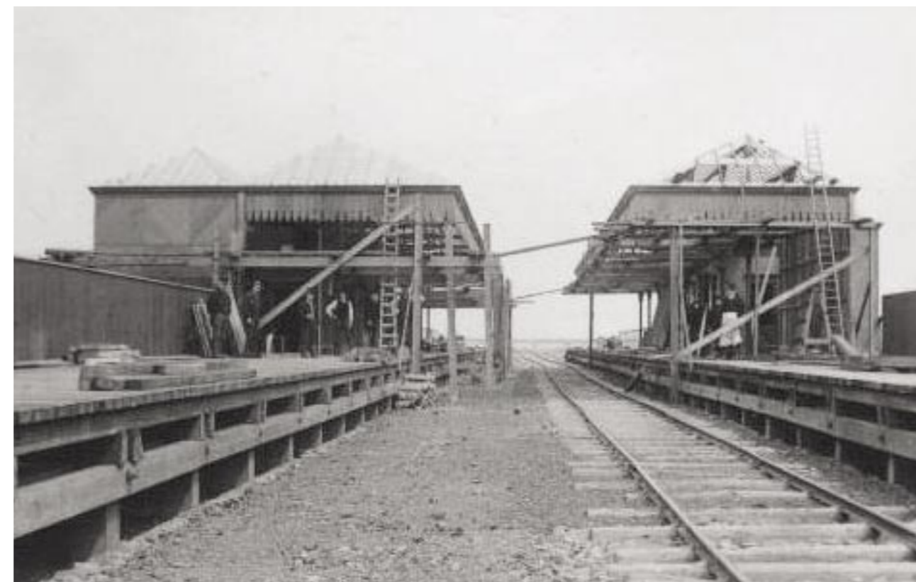
The area welcomes two new railway stations 20 feet higher than the originals.
