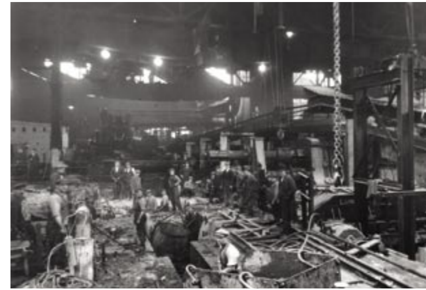
Following two years construction, the Partington Steel and Iron Company has finally commenced full production with blast furnaces and rolling mills becoming operational.
